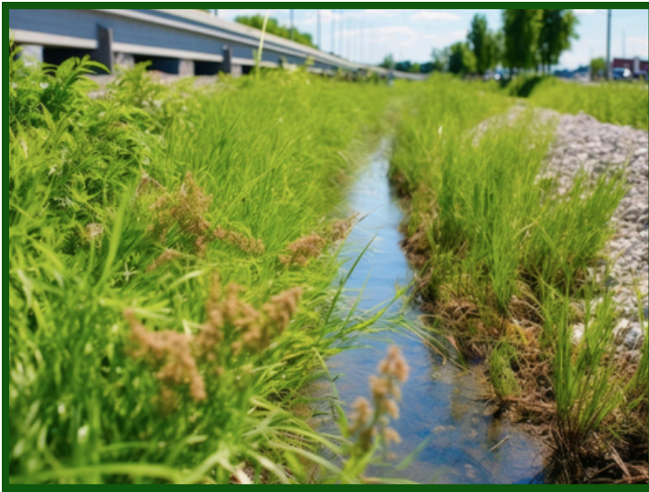
Left: An example of a swale with a wet base. Swales that contain vegetation are called bioswales (Newton, 2024).
