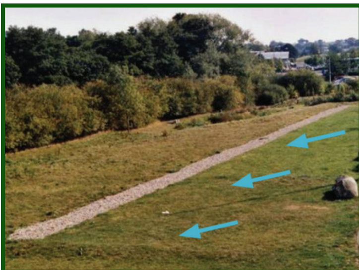
Left: The blue arrows denote a gradually sloped filter strip . This directs runoff to a filter drain and/or swale (Cambridge City Council, n.d.).
