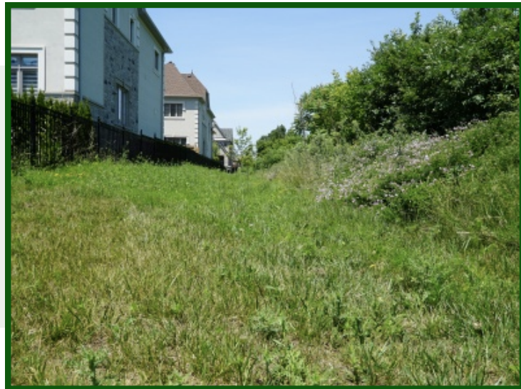
Right: An example of a swale with a dry base. Swales without planted vegetation are called grass swales (Sustainable Technologies, 2023).
